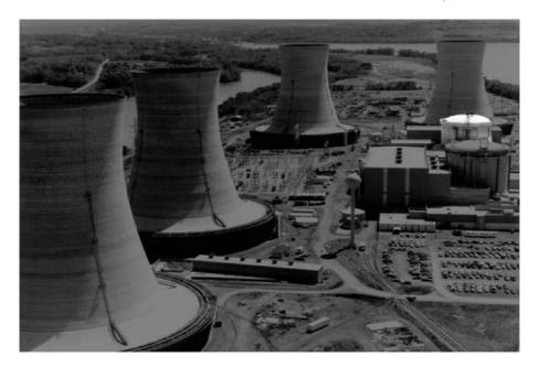
Department of Energy photograph of the Three Mile Island site. The reactors are located in the two small cylindrical containment buildings at the right center of the photo. Reactor 2 is highlighted. The four large hourglass shapes are cooling towers.
